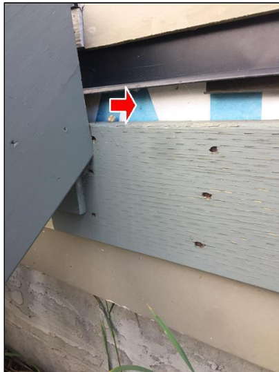
2.0 Figure 1(Picture) Exposed House Wrap
