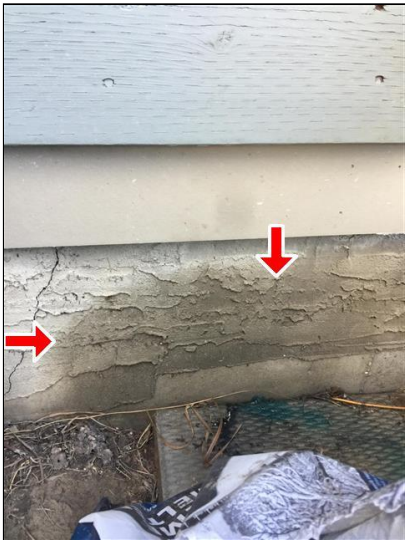
9.0 Figure 3(Picture) Moisture Foundation
