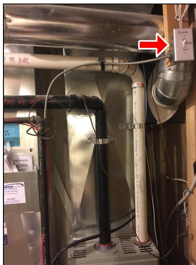
7.2 Figure 1(Picture) Furnace Shut Off
