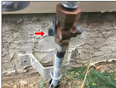
6.5 Figure 1(Picture) City Shut Off
