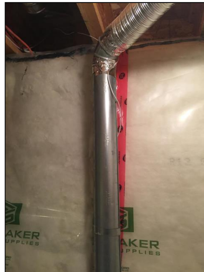
8.4 Figure 2(Picture) Extension Dryer duct
