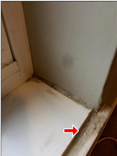
4.6 Figure 3(Picture) Wood Deterioration.
