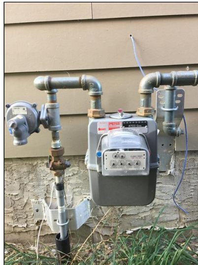
6.5 Figure 2(Picture) Gas Meter
