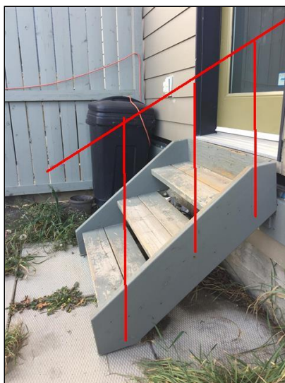
2.3 Figure 3(Picture) Missing Handrail
