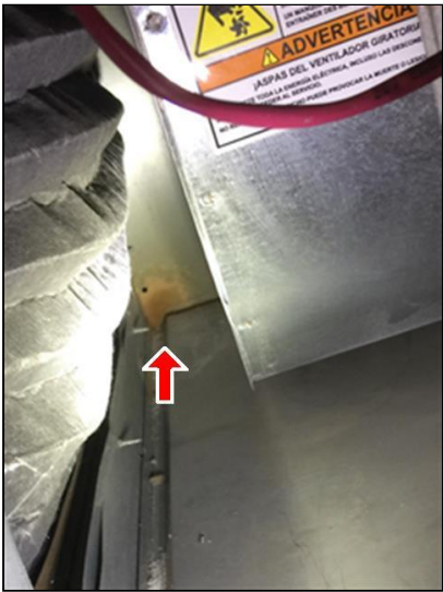
7.0 Figure 1(Picture) Corrosion in Furnace.
