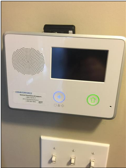
11.2 Figure 1(Picture) Main Security Panel
