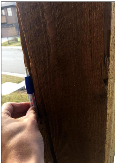
2.3 Figure 6(Picture) Comparison Crack
