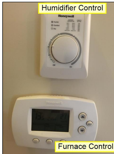
7.1 Figure 1(Picture) Furnace Control
