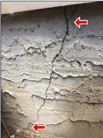
9.0 Figure 1(Picture) Foundation Crack
